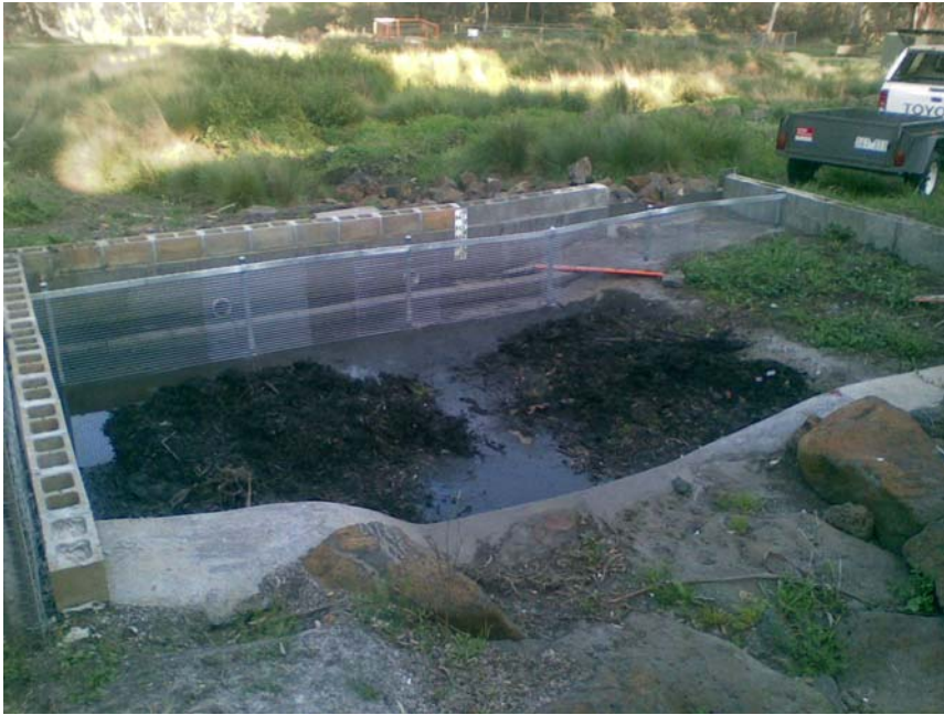
Figure 4.5 Example of primary treatment constructed to reduce blockage of downstream monitored pipes and diversion weir. In this case, the litter fence required monthly-cleaning to maintain satisfactory operation. Source: Peter Poelsma (University of Melbourne).
