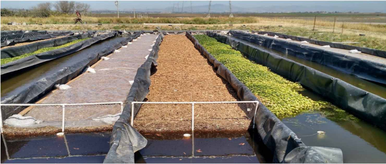
Figure 1 | Multi-chamber treatment system layout including source pipe and v notch in the background and white PVC drain pipes in the foreground. Other treatment reduction rate estimates are ongoing.
