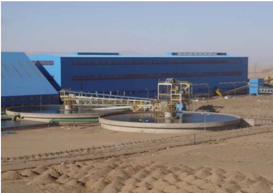
Figure 2 | Concentrator and thickeners.
